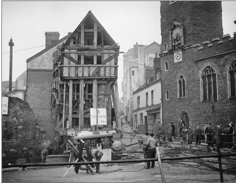
The installation of the house on the corner of West Street.
